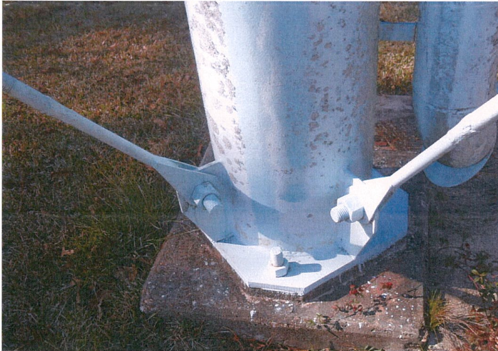
Figure 3. Condition of tank support foundation
