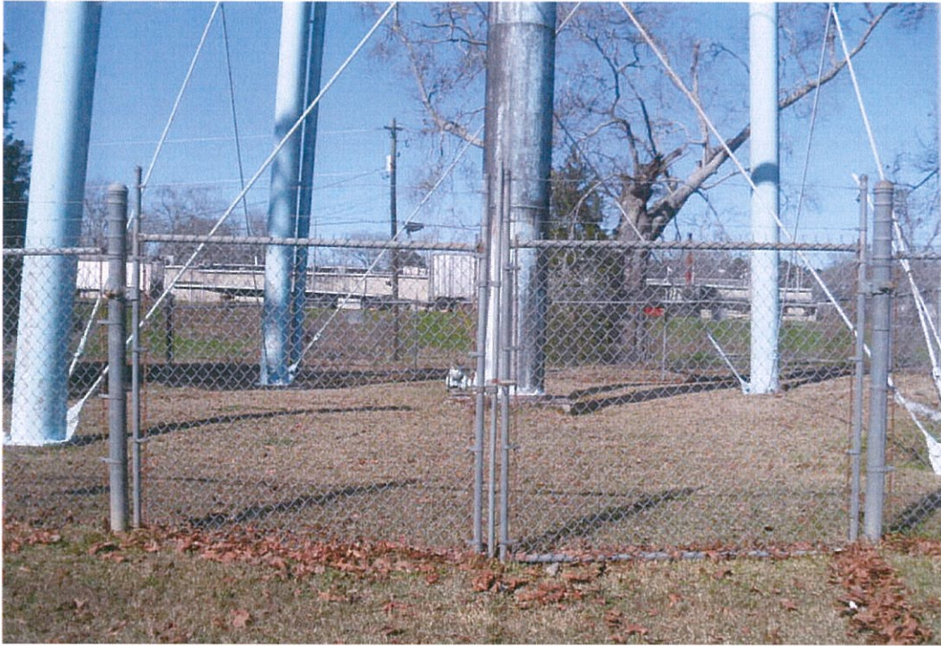
Figure 1. Locked entry gate
